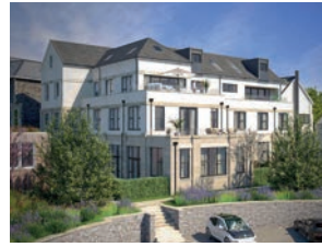
The Science Building.
